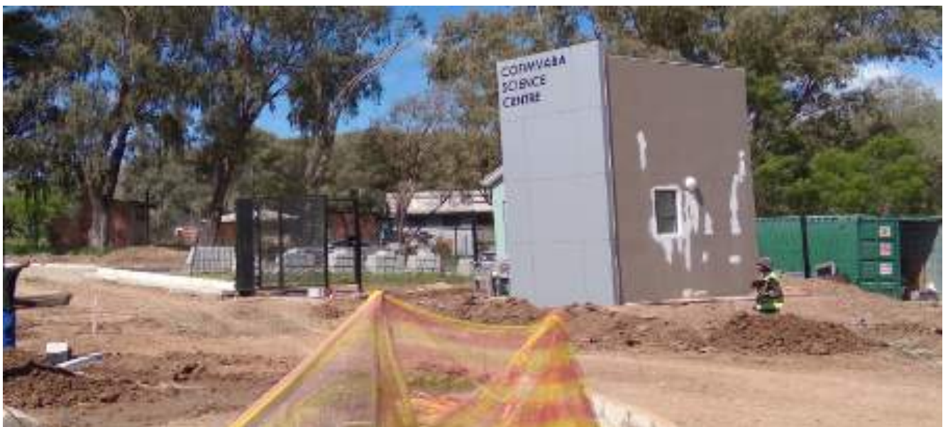
Figure 55: Entrance to the Science Centre, still under construction in December 2020
