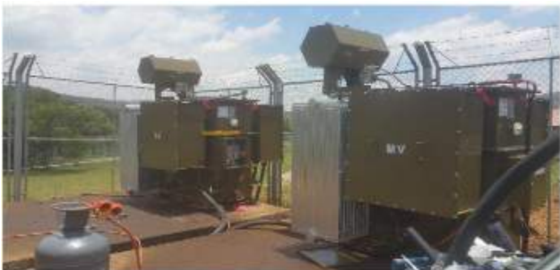
Figure 49: Installation of U –Bus Transformer
