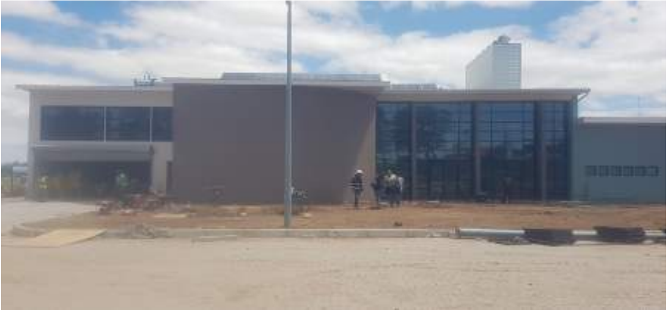
Figure 56: A view of the Science Centre from the parking lot (December 2020)
