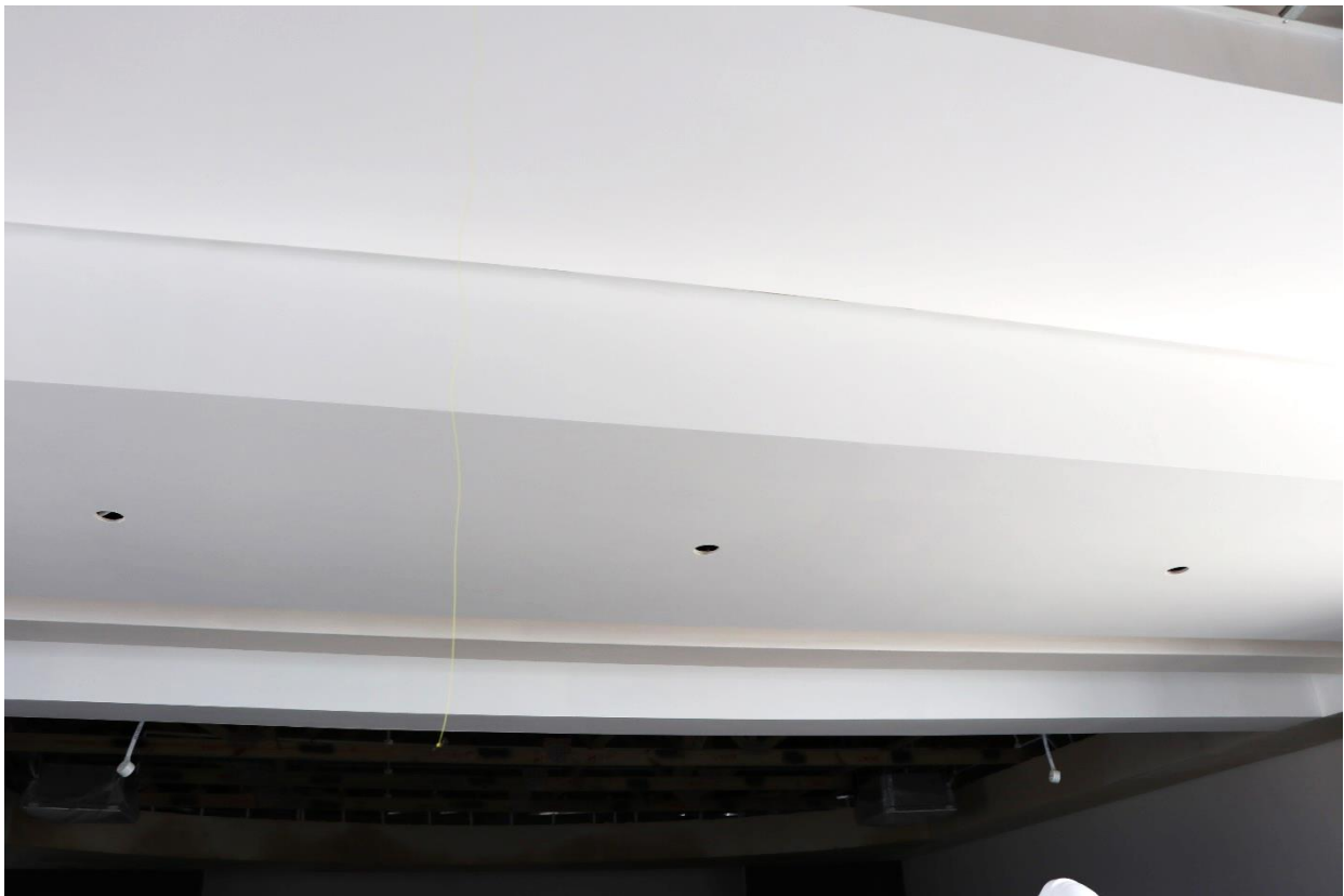
Figure 7 Bulkhead outside of Control Room
