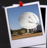
Polarisation: Linear and Circular Dish diameter: 9m
