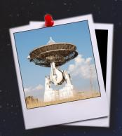
Slew rate: 10°/sec Dish diameter: 10 m Tracking mode: Program and
