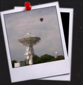
Slew rate : 3°/sec Dish diameter: 7.3 m
